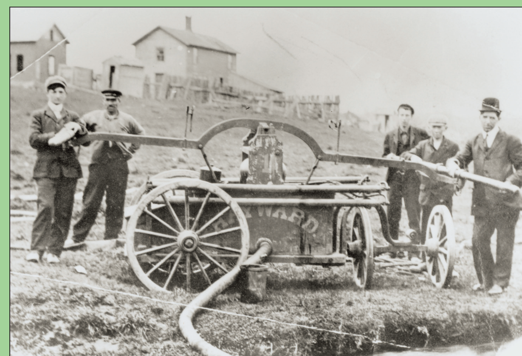
Hayward water pump for fighting fires
